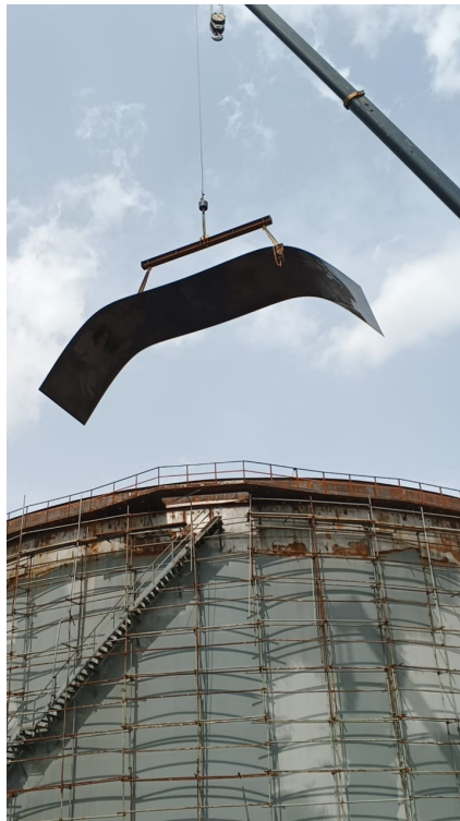
Crane lift of roof panel section
