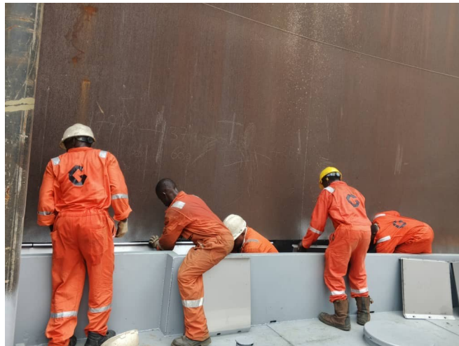
New floor plates being installed
