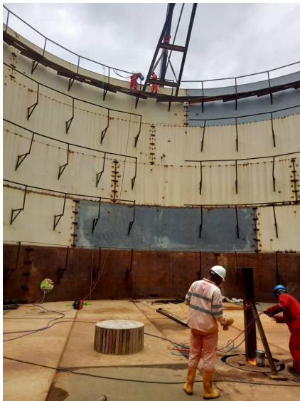
Roof rafters and centre column
