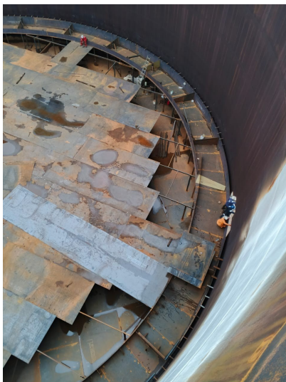
Aerial view of tank floor works
