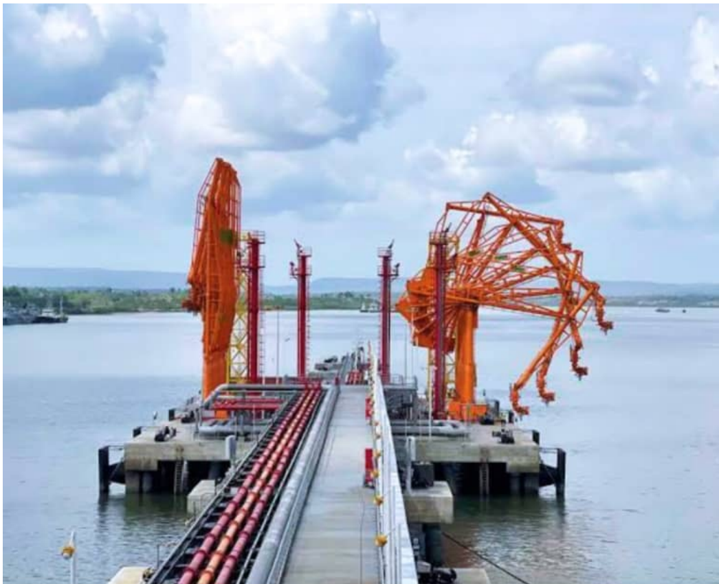
Twin loading arms on jetty platform
