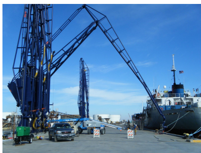
Loading arms under installation
