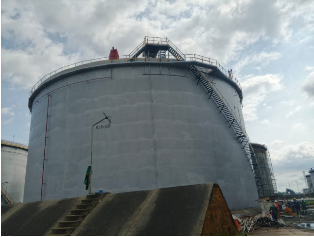
Completed tank 52TK57D
