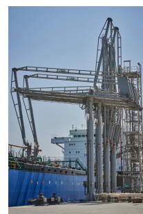
Loading arm walkway & structure
