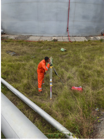
Pre-work site survey
