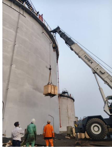
Materials hoisted to tank roof
