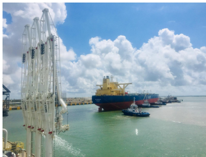
Marine loading arms at berth
