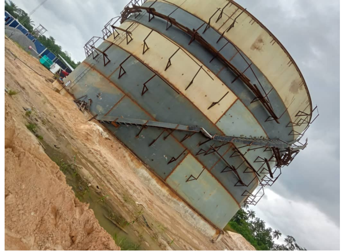
Roof structure works
